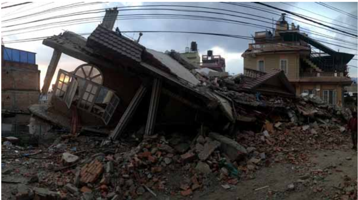
House after the earthquake
